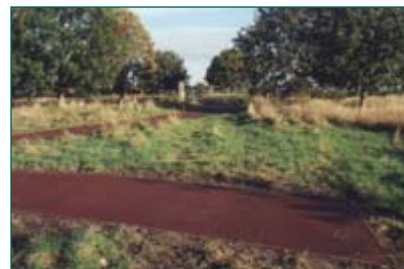
The new wheelchair path in the nature trail
